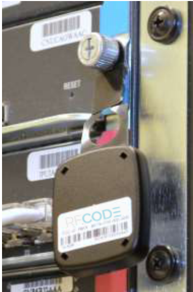
Figure 16: M174 tag mounted with thumbscrew tab secured
