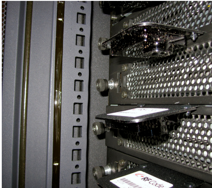
Figure 19: R104 Rack Tag Mounted with Lens Pointing Downward
